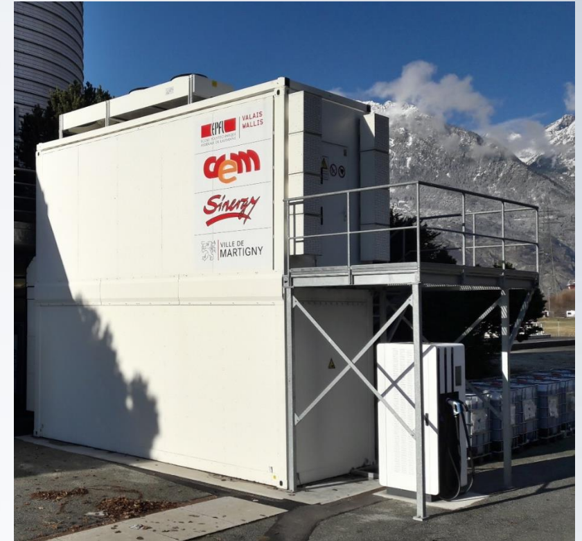
200 kW / 400 kWh Vanadium Redox Flow Battery connected to a 80 kW charger in Martigny
